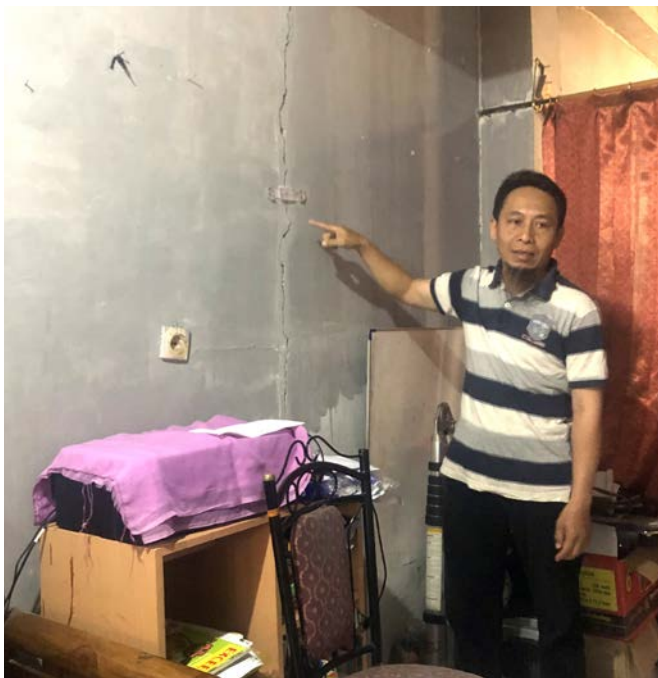
Villagers shows documented cracks in his house which were caused by the speedrailway tunnel construction
